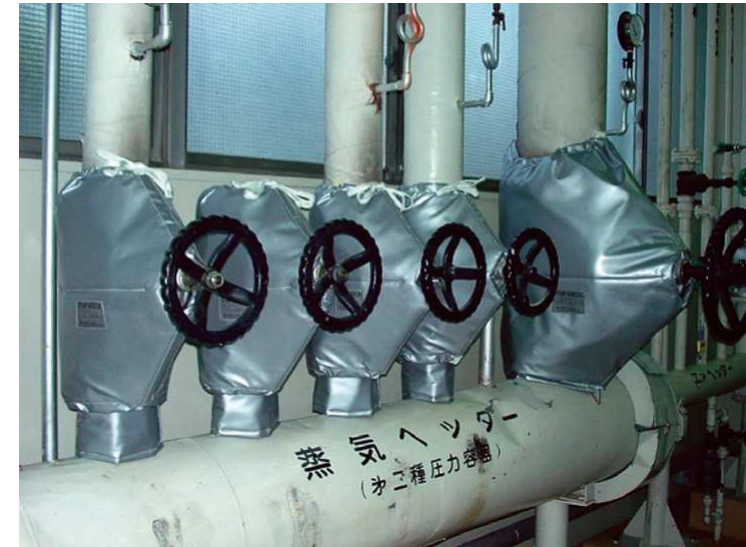
Heat retention of valves at the steam header
