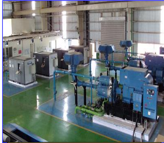
Screw Compressor With VFD Savings 250 MWH/Yr
